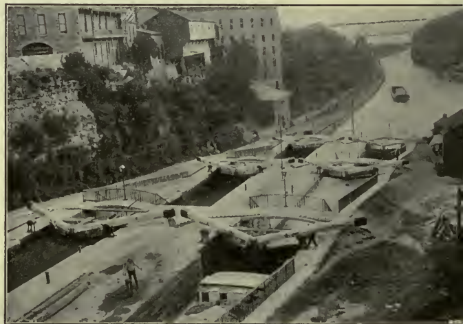
FIG. 184. — Locks in the Erie Canal. The canal boats are drawn into one of these spaces, which is then filled with water, raising the boat to a higher level. This is then repeated until the boat is raised to the level of the canal above the locks. Or, if a boat is going the other way, it is lowered in the locks by letting the water run out.
